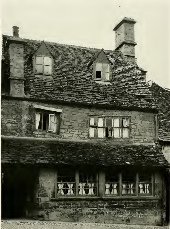
OLD BUILDING AT BIBURY The windows of the second story dip gracefully
